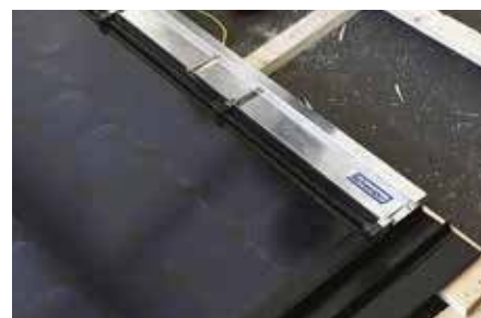
3 Fix the next rows of mounting clamps using the mounting gauge.
