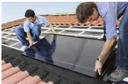
2 Insert modules from right to left and from bottom to top.
